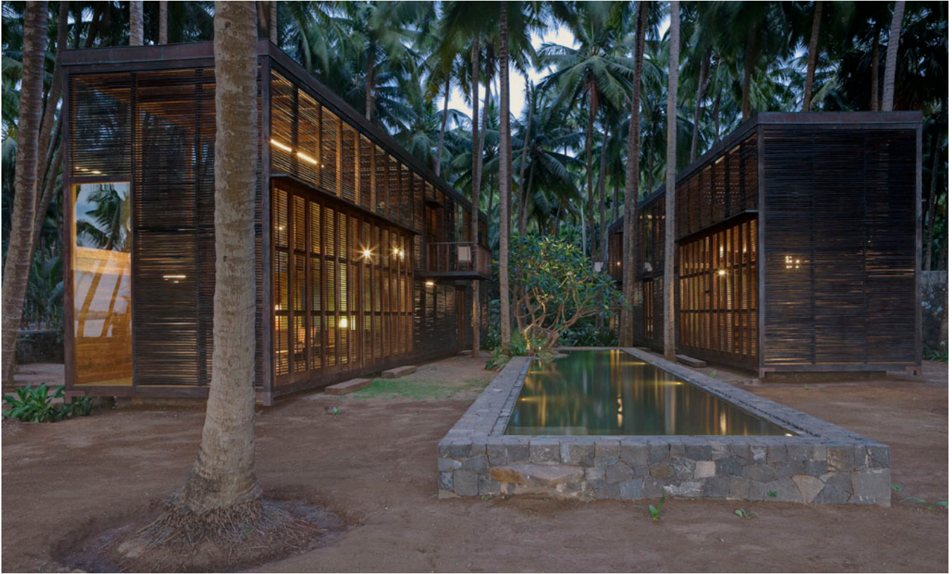
View from the West of the North and South Blocks with the pool in the middle lit in the evening.
