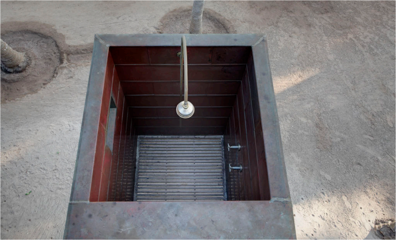
Top view of the hanging shower area of the Master Bathroom with copper plates used on its surface.
