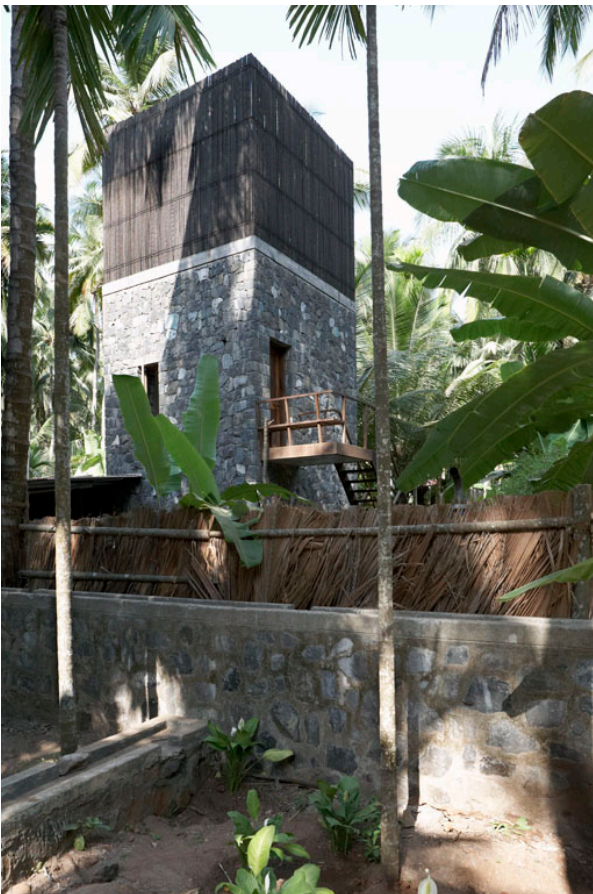
View of the camouflaged storage water tank raised on a stone structure.
