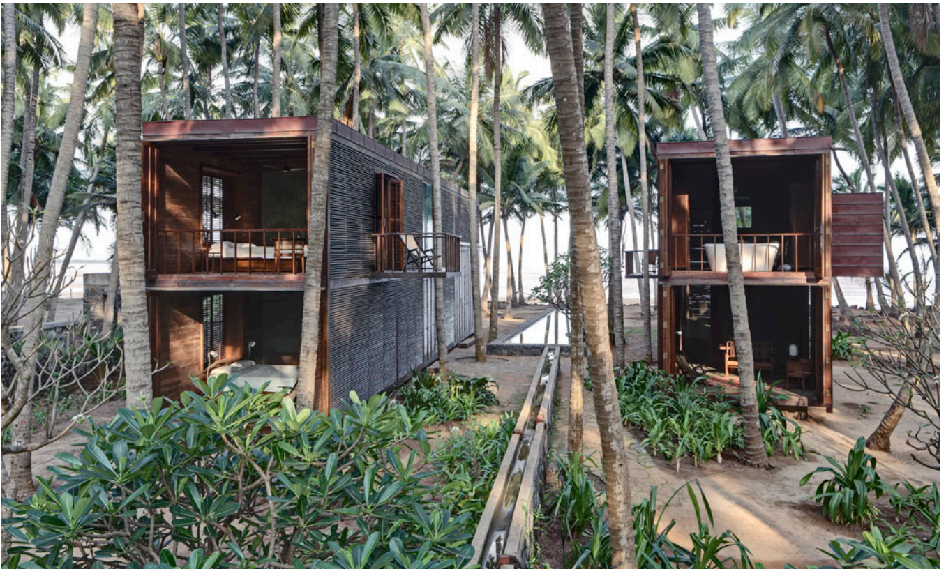
View of the two blocks from the east side showing aqueduct and pool in the centre. North block shows study and master bathroom while the South Block shows two guest bedrooms.
