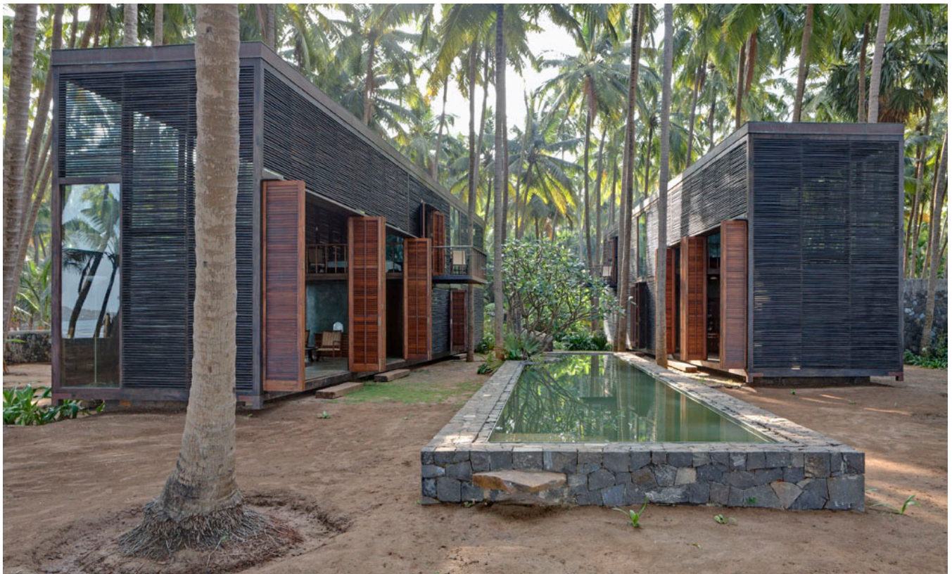
View from the West of the North and South Blocks with the pool in the middle and coconut plantation in the background on the East side of the plot.
