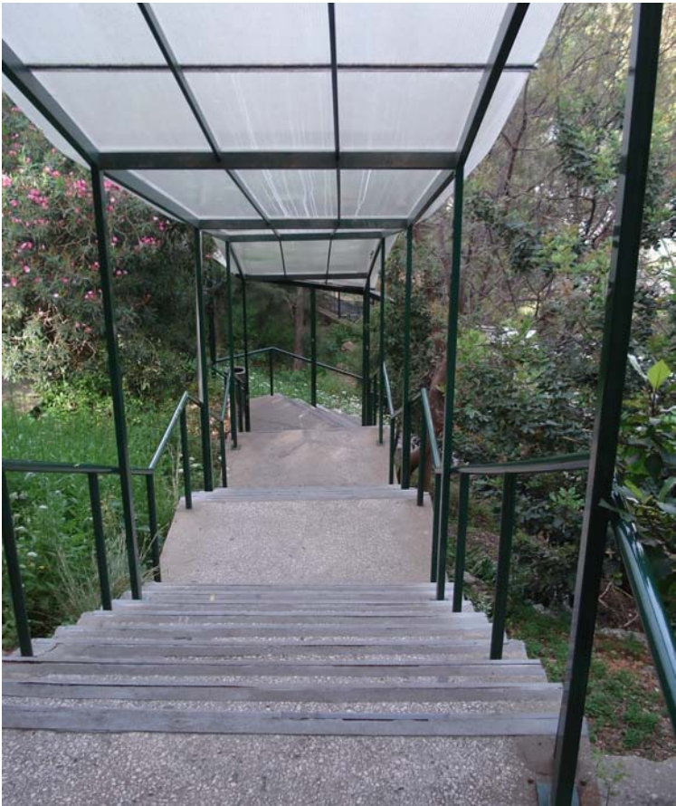
Stairs linking the different levels of the campus.
