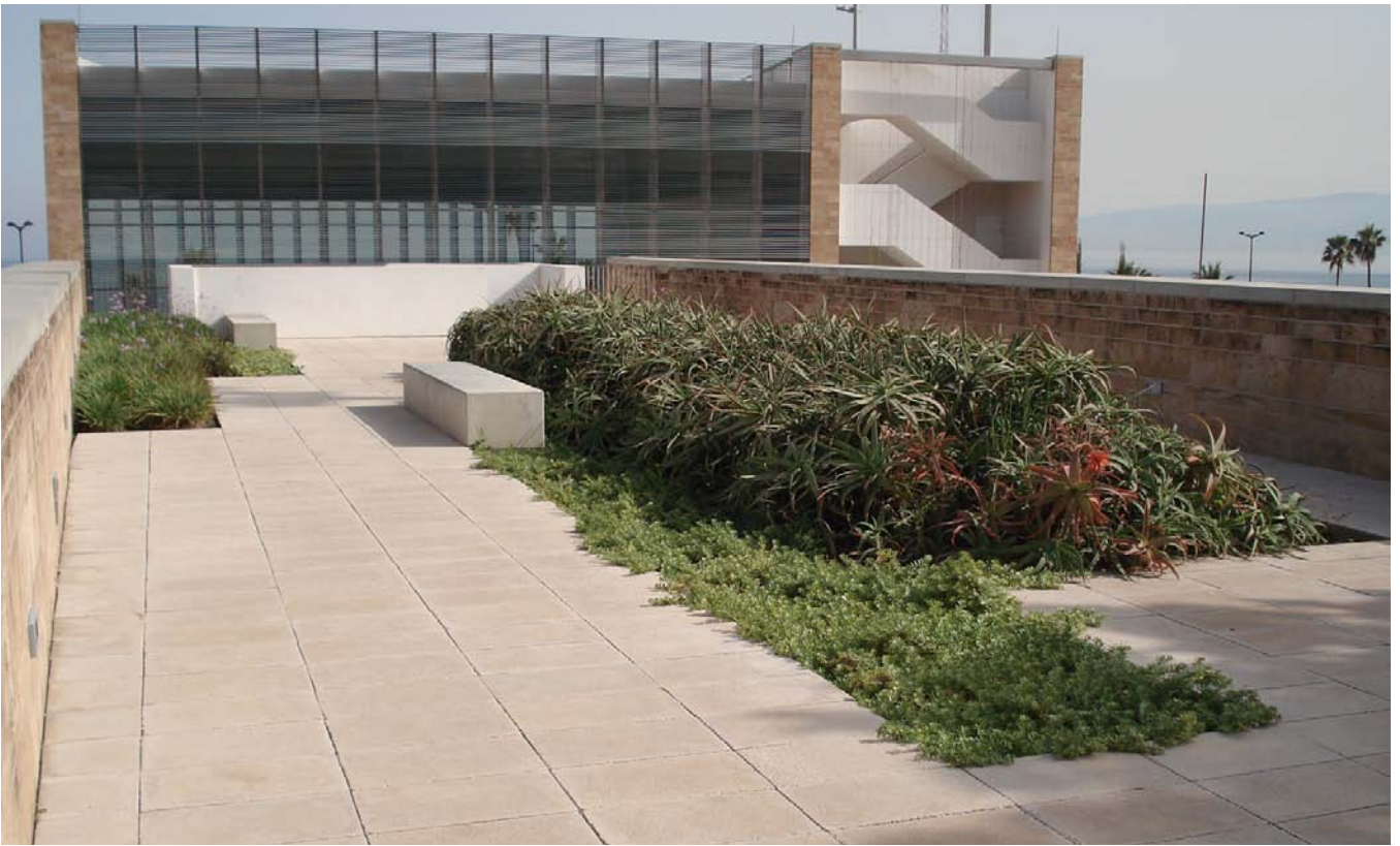
East façade of the Charles Hostler Student Centre.
