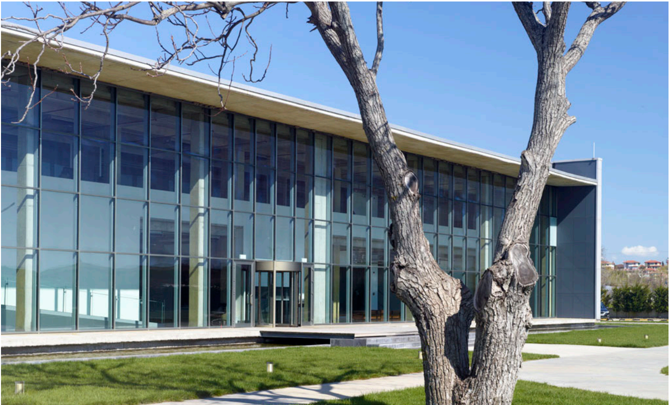
North view of the façade.
