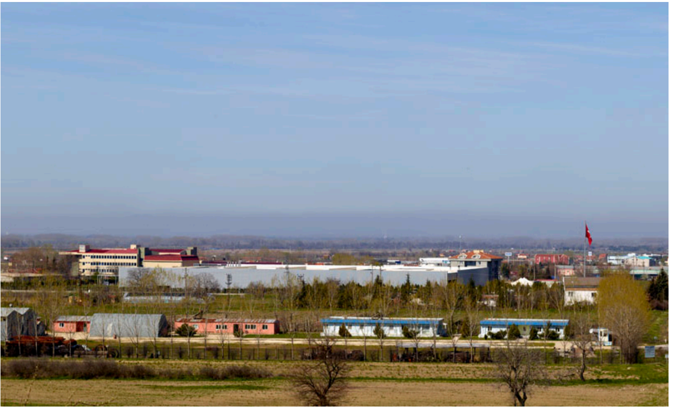
General view of the site.
