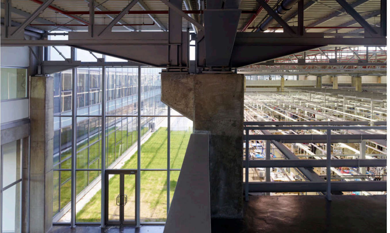
View of the production hall from the first floor.
